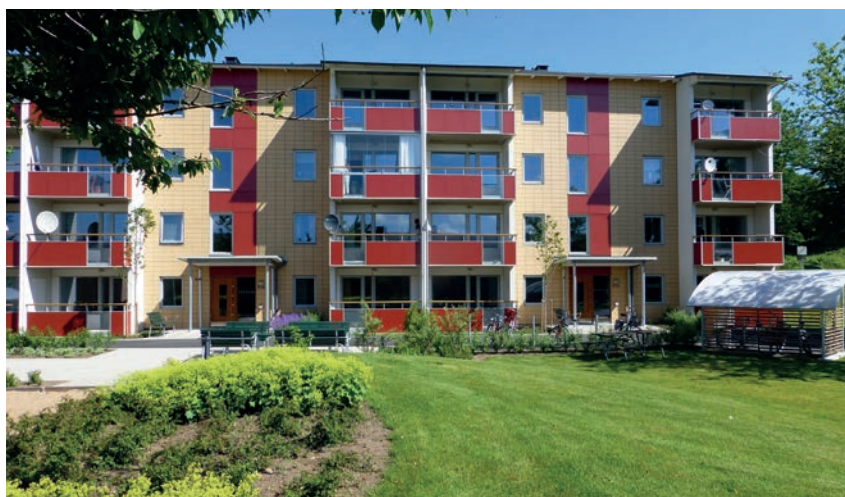
Retrofitted building in Sweden
