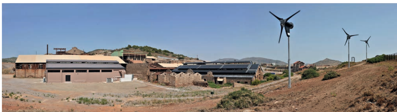
View of the Lavrion demonstration installation
