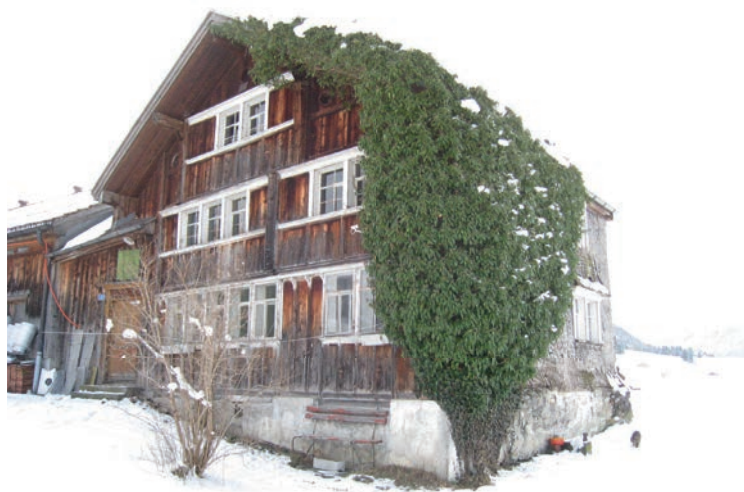
This typical alpine “Strickbau” is being retrofitted within 3ENCULT
